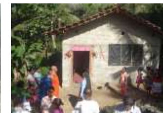
Newly Built Home (April 2015)
